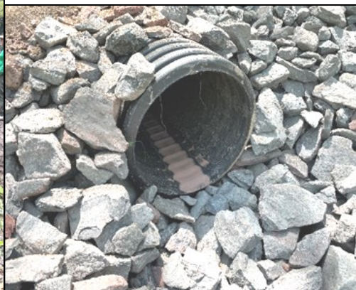
Photo L-R: Installation of new cross pipe, cross pipe outlet with stabilization, and finished DSA surface.
