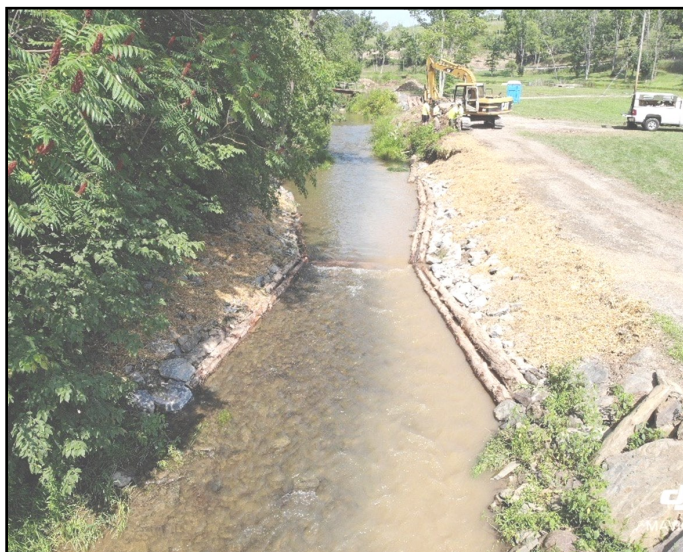
Photo: A log-framed cross vane installed in Hemlock Creek at the Moore property as part of a fish habitat improvement and streambank stabilization project completed this summer in Hemlock Township.
