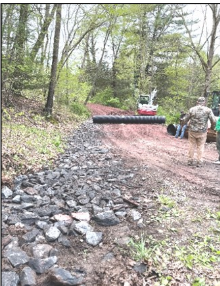
Photo L-R: Installation of new cross pipe, cross pipe outlet with stabilization, and finished DSA surface.
