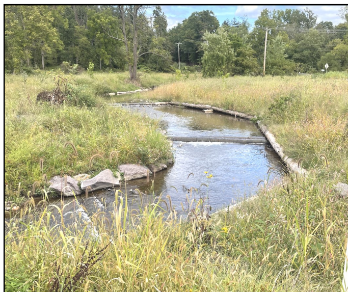
Photo: Stream structures and shrub/pollinator buffer for erosion control and fish habitat installed on East Branch Briar Creek, Berwick.
