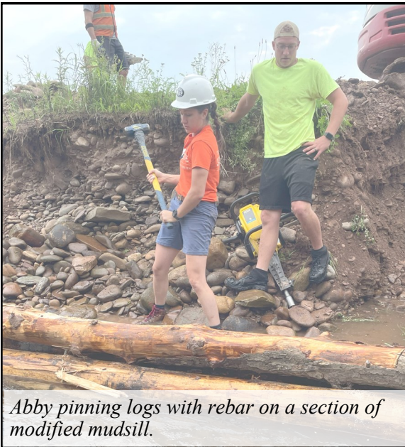
Aaron drilling holes to pin face logs together on a section of modified mudsill.
