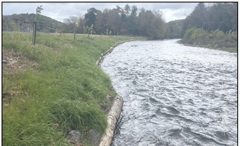
Before and after images of a section of Fishing Creek in Benton Township. 520 linear feet of modified mudsill and a 50-foot wide buffer were installed this summer.
