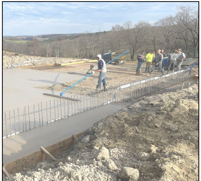
Workers pour the floor of a manure storage structure funded by a National Fish and Wildlife Foundation grant, Benton Township
