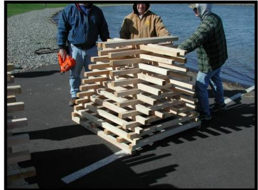
Placement is traditionally accomplished by specially equipped boats during softwater periods (no ice). Submerged structures are normally placed in a row with 4' to 8' spaces between individual structures. Normally 10 to 20 Porcupines are placed at one site. Structures are submerged in 10' to 15' depths (Lynch, Johnson & Kayle 1988) (Lynch, Johnson, Durfey 1988) along the contour parallel to the shore.
